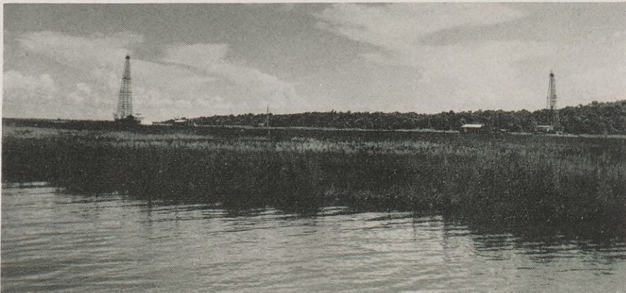
Weeks Island was pushed up from the southern Louisiana marshland by a salt dome. Completed wells and drilling rigs circle the island's outer rim.
