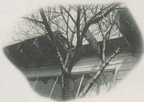
Rather than destroy this tree, Echols cut a space for it to grow through the eaves.
