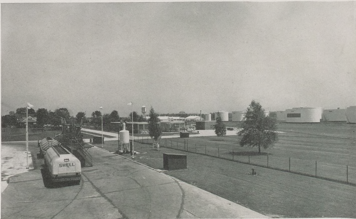
At Zionsville Pumping Station and Terminal (above) there has been an increase in Shell products received daily from Wood River due to the greater capacity of the East Line made possible by the installation of the four new remote control booster stations. From here a portion of the products are pumped on to Muncie, Indiana, and to points in Ohio.
