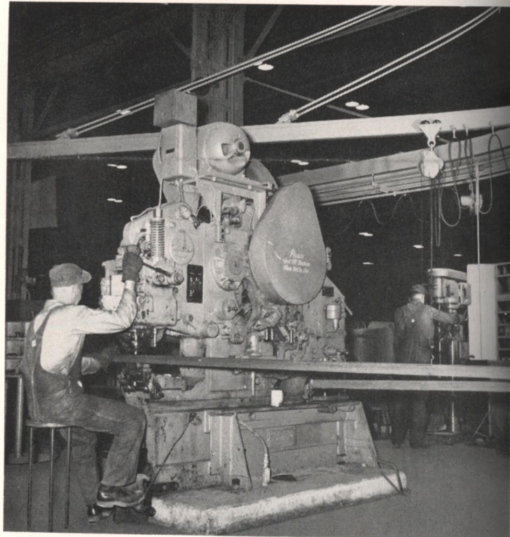
C. D. Elliot, foreground, operates a punch and shear machine, which shears 8" x 8" angles 1/2" thick. W. L. Calhoun reams exchanger baffles in background.
