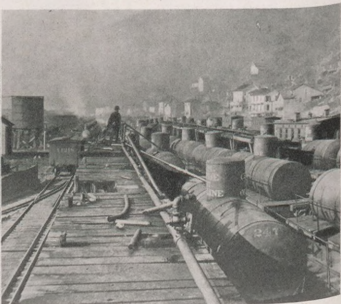
Iron boiler tank cars of the 1880's, capacity 85 barrels each, were forerunners of today's modern tank car fleets. Pipe lines, often laid along the surface of the ground, fed the tank car loading racks.
