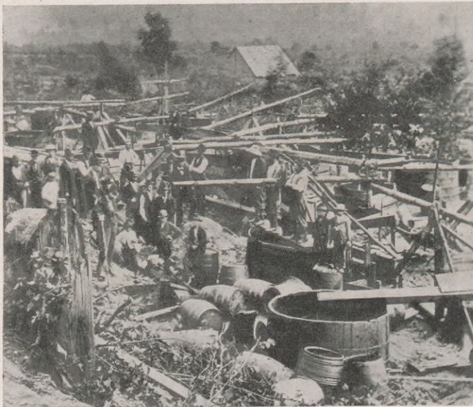
Grasshopper Wells, near Titusville. Only 17 feet deep, the 13 wells in this section produced 100 barrels of oil per day.
