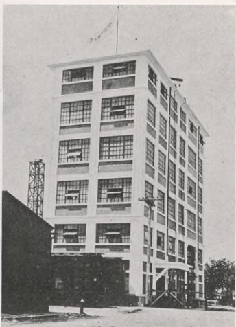
Liberty Bell Flour Mill, San Antonio, Texas, where Texaco Ursa Oil is being used on all shaft bearings, as well as for lubricating the Bush-Sulzer Diesel Engine
