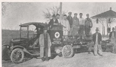
Telegraph and Telephone construction gang building new line between Sherman, Texas, and Healdton, Okla.
