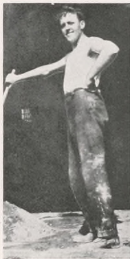
Construction Foreman Jas. H. Dickson in action at Attleboro Mass. Station
