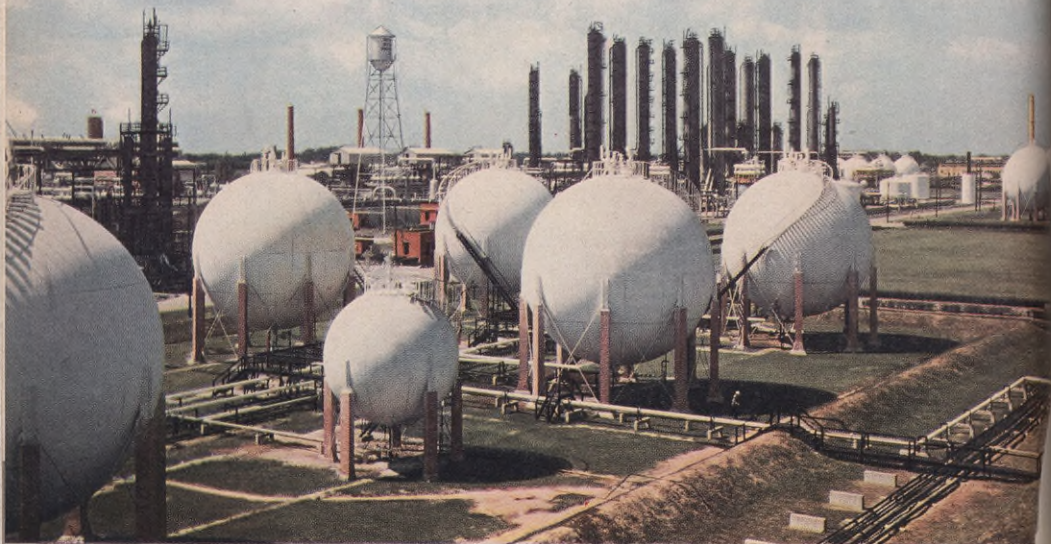
A PORTION OF NECHES BUTANE PRODUCTS COMPANY, LARGEST BUTADIENE PLANT IN THE WORLD
