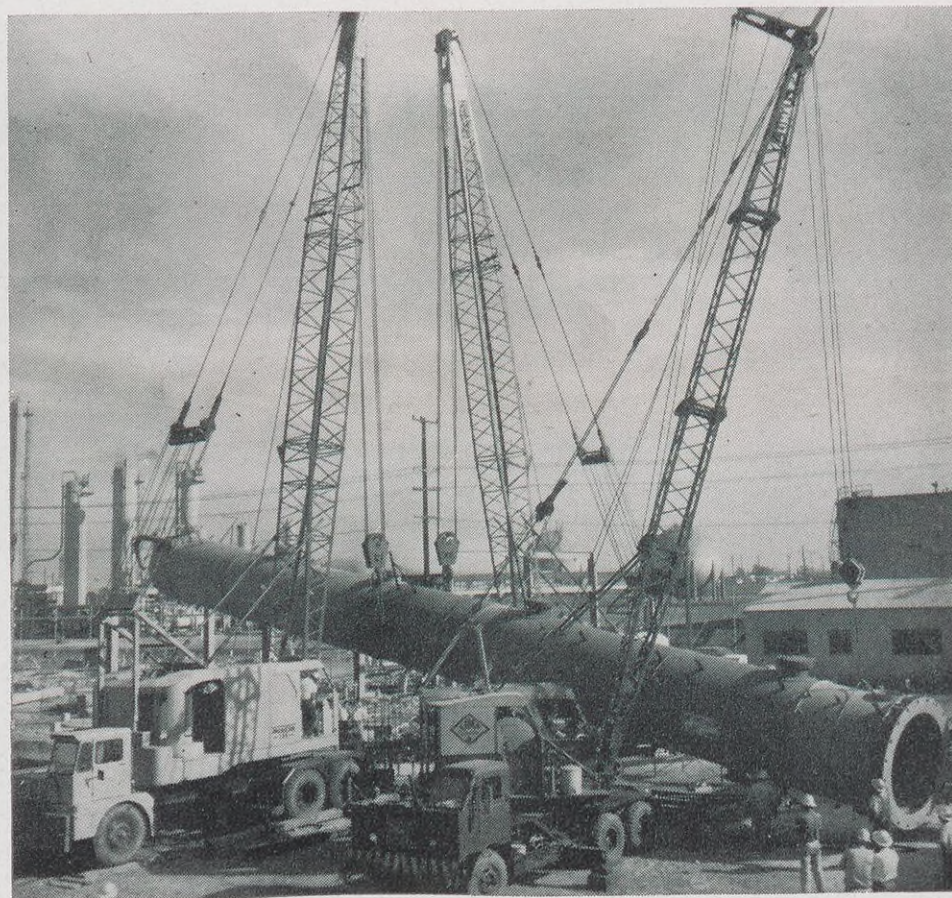
Most refinery expansions of Shell and other oil companies, such as this platformer-desulfurizer unit being built at the Wilmington Refinery, are to improve products. This unit will manufacture high octane gasoline. But while the price of gasoline (excluding taxes) went up only 12 per cent from 1947 to 1958, the cost of constructing units such as this one at Wilmington went up about 62 per cent.
