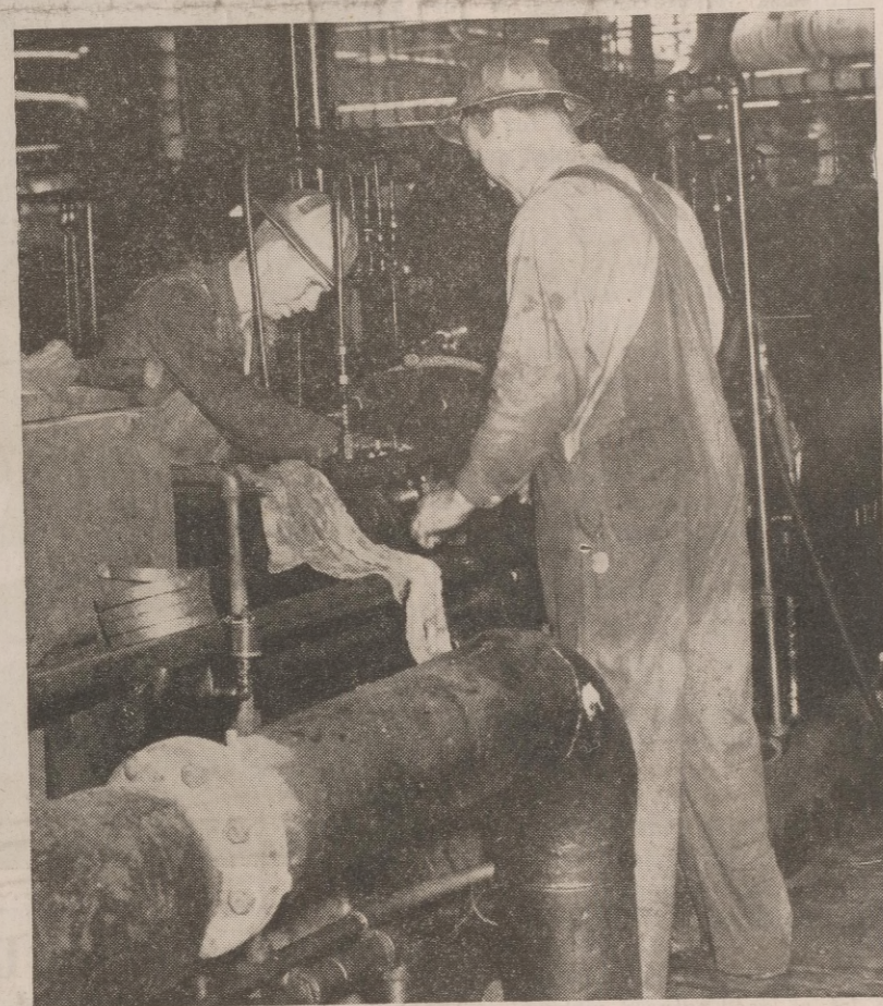
Steam engine stuffing box of huge charge pump at Dobbs 9 reform furnace is repacked by machinist C. E. Bergfeld, right, and helper L. F. Cain.
