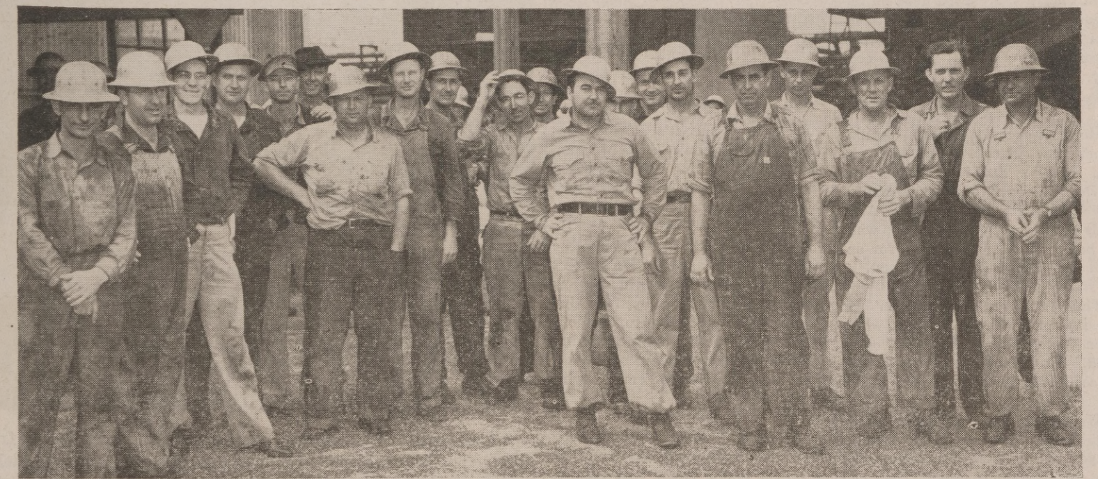
The Pipefitting craft is the largest in the refinery and to it falls the job of removing and installing all pipe which, even the layman can see, is a tremendous job. Assembled here following a day's work are a few members of the craft. Faces discernible are, left to right; B. M. Gillum, G. E. Butler, J. M. Willard, W. C. Richardson, O. J. Clements, C. A. Russell, L. G. Utecht, W. E. Stagner, L. C. Presswood, H. F. Ireton, R. E. Cunningham, J. E. Martin, B. N. Stubbs, M. C. Roberts, J. K. Bryant, J. S. Morris, N. G. Parten J. T. Kennedy, E. Duke, and W. M. Bostic.
