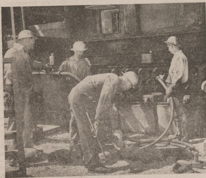
Specialists in the cleanout of units is four Cleanout men at reforming furnace. Removing tube cleaner from a cleaned tube is F. Wetuski, right. Mike Robinson, left, D. R. Dowdy, operate power. A. Canady (side to camera) lifts return bend which will connect two of the tubes.
