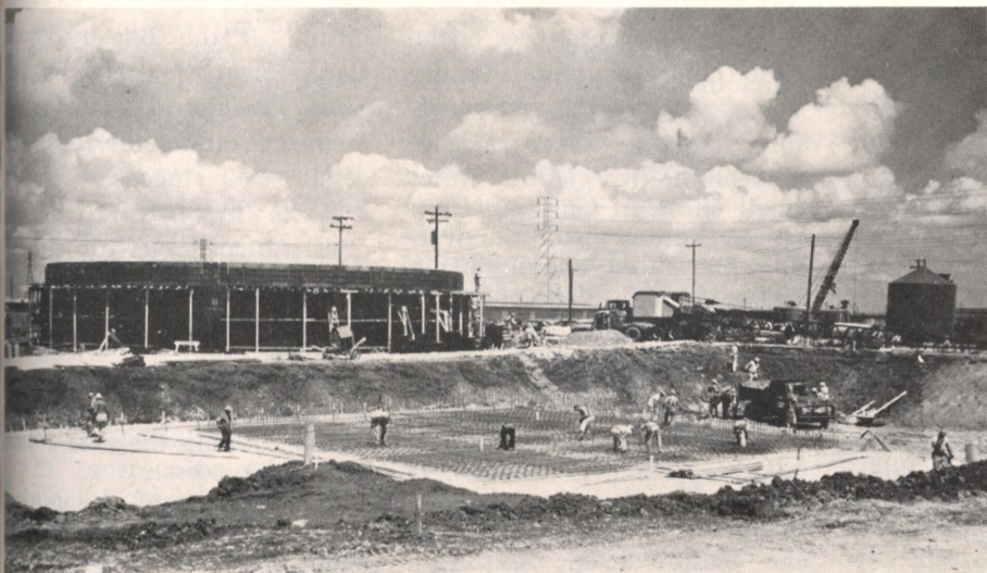
The water treatment plant, undergoing construction, is shown in the background
