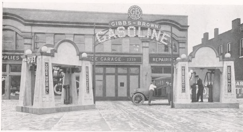
Gibbs-Brown Filling Station, St. Louis—Self-measuring pump system of handling gasoline
