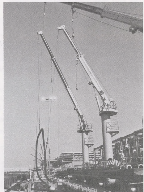
IT'S OFFICIAL NOW...Newly constructed DPMC Dock 3, shown here shortly after it began operating in November 1987, recently was the site of a dedication ceremony held in its honor. Attending the ceremony were Dock employees, their spouses and families, Coast Guard representatives, and DPMC and Head Office management.
