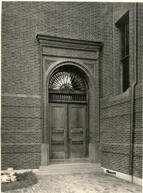
Plate XVI. Robert Gould Shaw School—Detail of Entrance.
