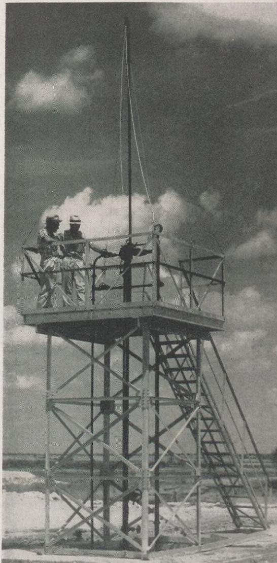
Shell Pumper E. B. Wilkins, right, above, and a service company representative survey well head equipment mounted on a 12-foot steel tower where it is accessible even during floods.
