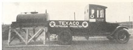
Combination Truck with Sliding Rack for Delivering Drums and Tins
