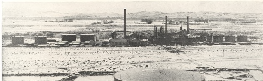
New Refinery of The Texas Company at Cody, Wyoming
