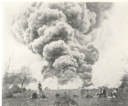
Tank Struck by Lightning near Titusville
