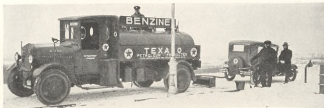
Tank Truck Being Filled at Amsterdam Bulk Station
