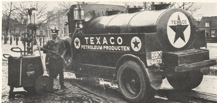
Three Thousand Liter Tank Truck Delivering Gasoline to Wheel Tank
