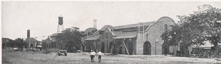
Tampico Works—Shop building at right—Power house at extreme left.
