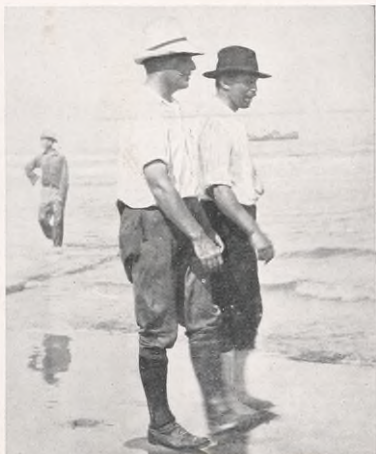
D. J. Moran, General Superintendent of Construction in Mexico, and T. Reiber, Assistant Superintendent of Port Arthur Works, when they were getting out the sea-loading pipe lines.
