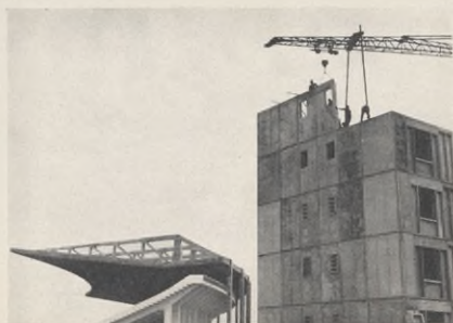
Prefabricated wall slabs are fitted at Casablanca ▶ apartment house project.
