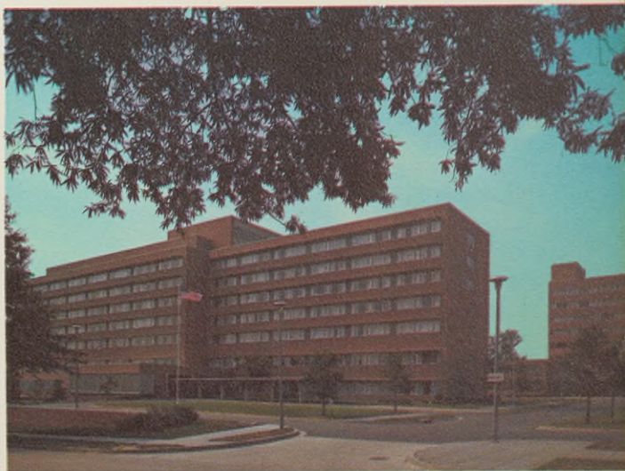
Hot Shoppes provides food service for both patients and staff in the 300-bed Sibley Hospital in Washington, D. C.
