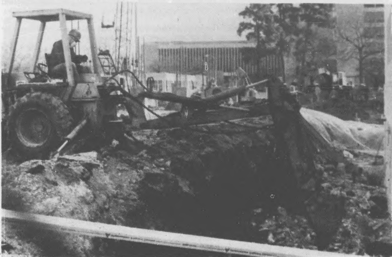
WORK CONTINUES ON LIBRARY EXPANSION PROJECT
