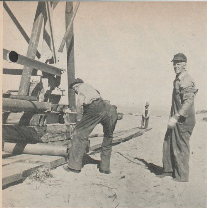
The board track over which the derrick was walked.
