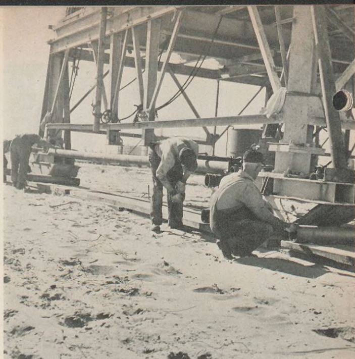
Placing rollers under substructure as derrick moves forward.
