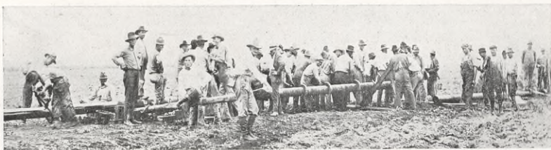
Pipe Line Connection Gang between Bridgeport and Fort Worth
