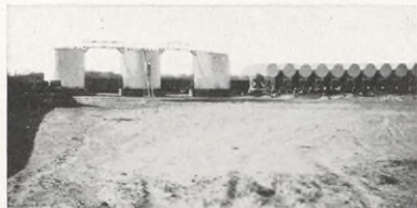
Equipment of storage tanks at Pueblo Station, Oct. 3, 1911
