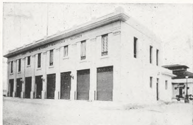
Garage and Shops The Sanitary Department of the City of Havana uses Texaco oils throughout.
