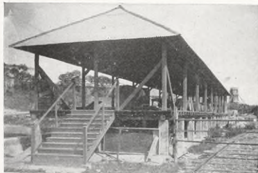
How the disinfecting oil is handled The Sanitary Department of the City of Havana handles much oil for disinfecting sewers, cess pools, etc., to prevent the propagation of mosquitoes. Bowser tanks with a capacity of 100,000 gallons are under the platform. The tank cars are discharged into these tanks. The distribution is made by tank wagons for the city use, and by steel barrels for outlying districts. Texaco "Paraffine Gas Oil" has proved the most satisfactory oil for this purpose as it has the spreading qualities necessary.
