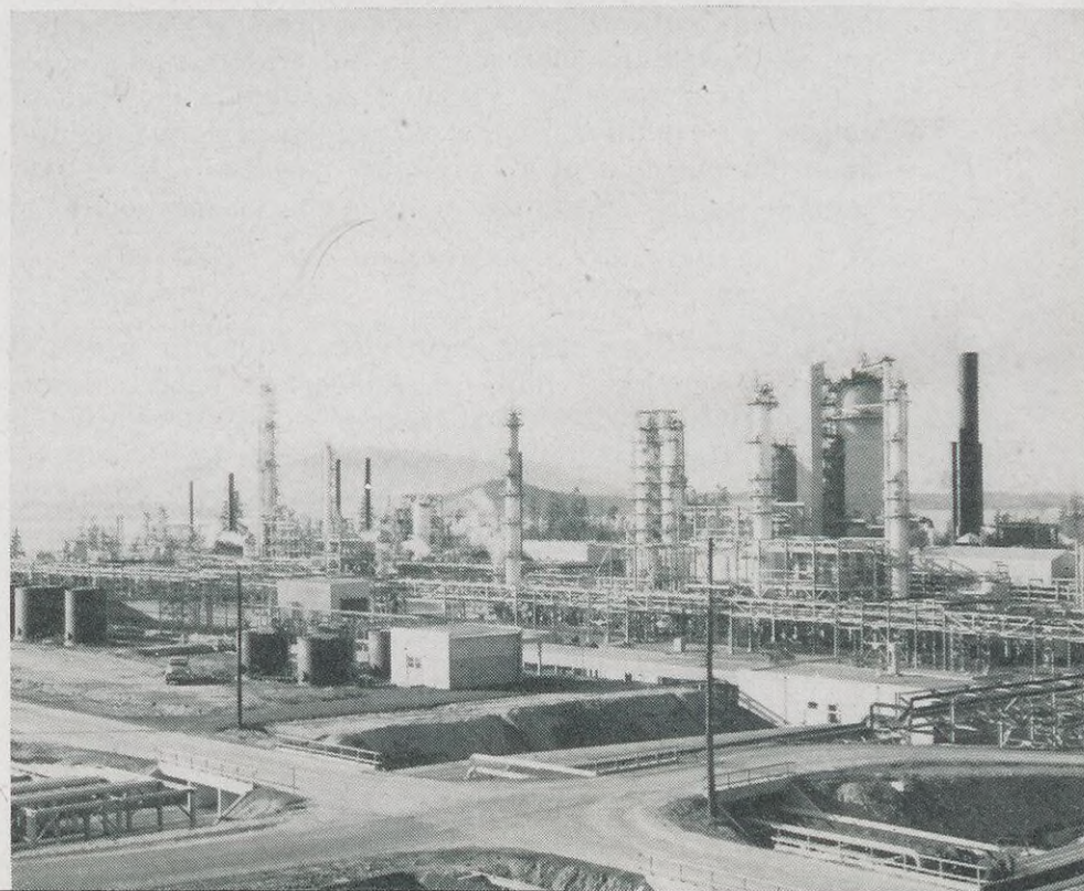
Shell installed the first two-stage catalytic cracking unit (the largest structure at right below) at its new Anacortes, Wash., Refinery in 1955.
