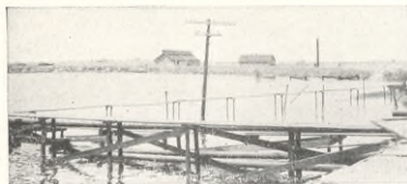
Artificial lake, Electra Gasoline Plant
