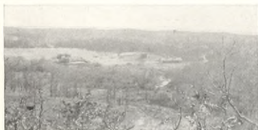
Youngstown, Okmulgee County, Oklahoma, Pipe Line Station
