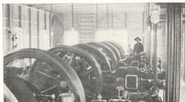
Compressors in one section of Gasoline Plant
