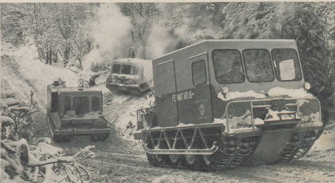
2. Shell seismic parties in the north country use "Bombardier" personnel carriers equipped with treads to move out of camp to the scene of the shooting. The caterpillar-like tracks are ideal for traveling over the muskeg, which will support vehicles only when it is frozen solid.
