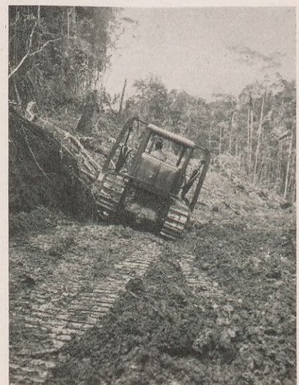
It's rough going in the Oriente, and building a road from Ayuy airstrip to the drilling site at Macuma takes skill with the bulldozer.
