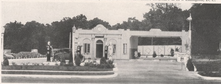
Texaco Service Stations are Found in 48 States of the Union. This Attractive Structure is in Washington, D. C.
