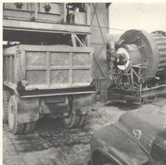
Asphaltic surfacing for Massachusetts Turnpike is being mixed in 4,000-ton batches at a plant served by Texaco.
