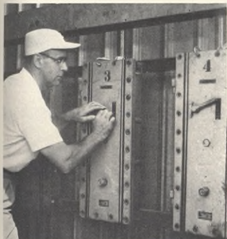
Switches on all electrical circuits leading to loading racks are quickly shut off.
