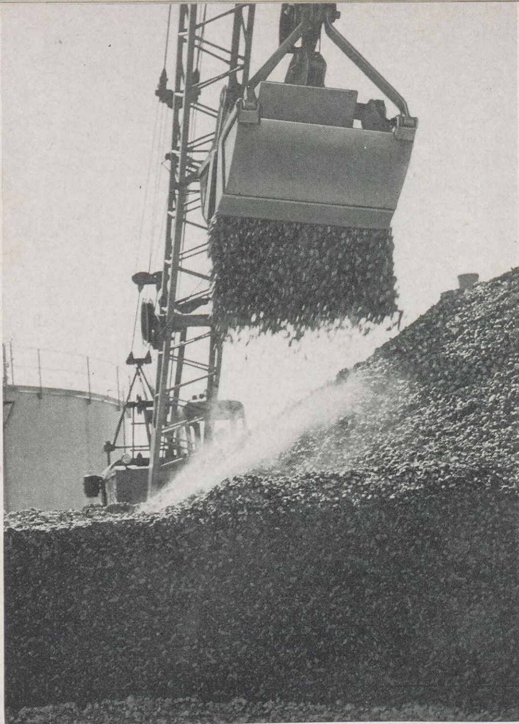
Clam shells , brought to the Shell Chemical Norco Plant by gondola car, are emptied by a crane and stacked near the two neutralizer pits.
