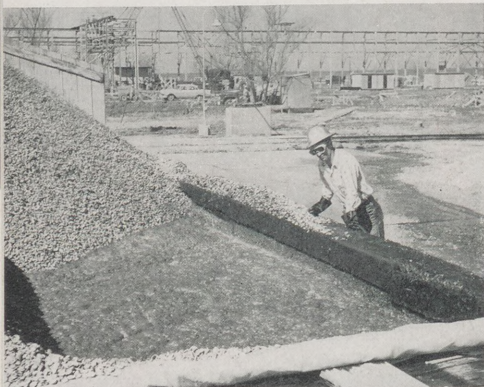
Operator M. L. Lauve watches as hydrochloric acid dissolves shells, resulting in calcium chloride.
