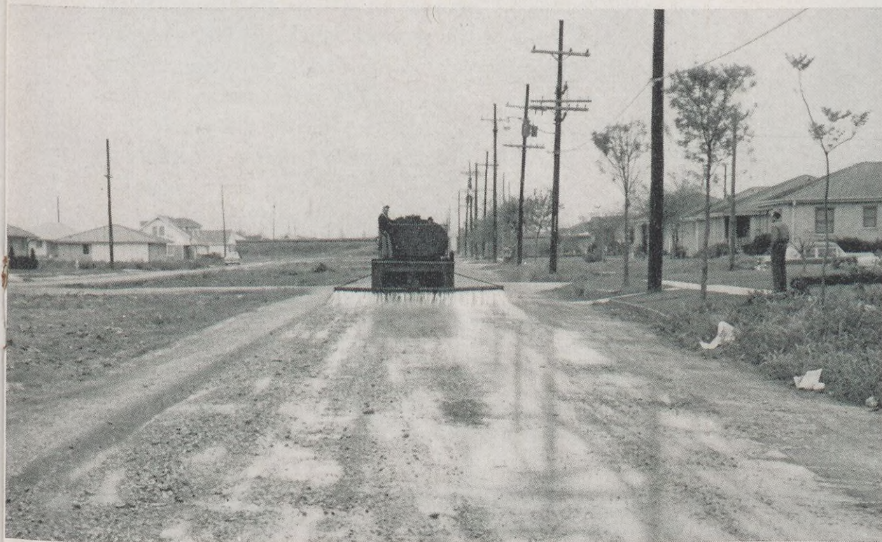
Calcium chloride sprayed on this New Orleans street by the truck in background keeps dust from forming by absorbing water from the atmosphere.
