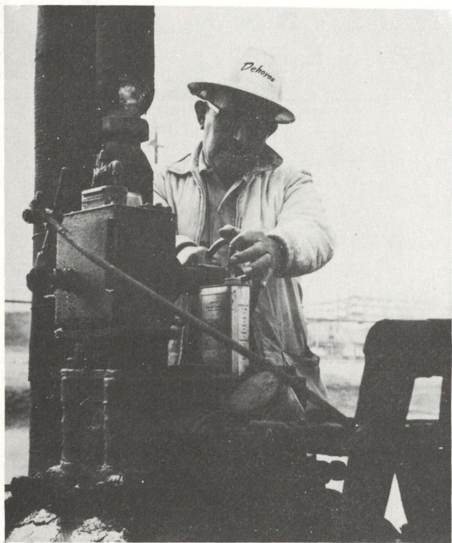
FISH PROTECTOR...on the waterfront. B. De Hoyos, Effluent Water Treater No. 1, adjusts the skimming pump control valve on a settling pond at the biofilter.
