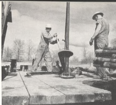
Converting an oil well to a water injection well is a basic step in the flooding process.
