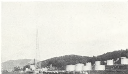
Tanks at Pryse Works
