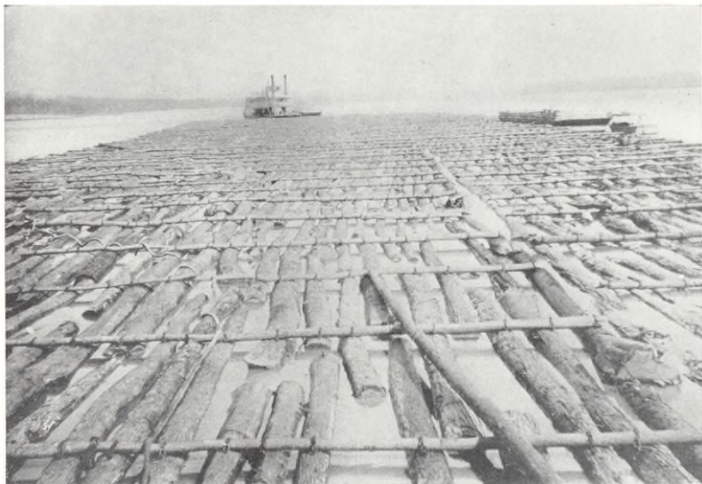
Tow of timber on way to sawmill
