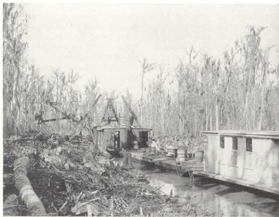
Dredging a canal for timber operations
