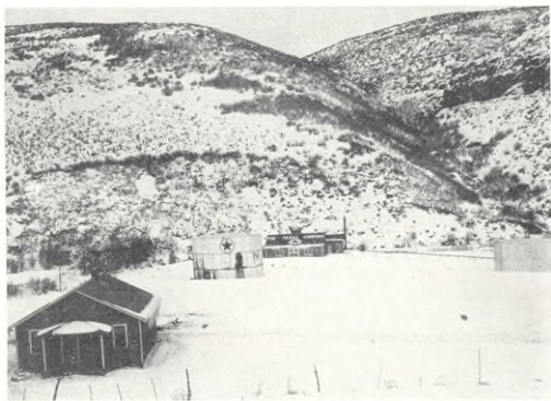
Solitary hillside pumping station a few miles from Craig
