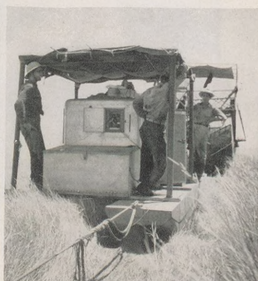
In some locations, seismic crews use both helicopters and marsh buggies. The aircraft (left) setting down near a marsh buggy track is used by men who set out and recover seismometers. The cumbersome marsh buggy (center) tows shooting and recording equipment to the proper locations in the marshes. At right, crew members stand by the seismic recording instrument as they await the detonation of an explosive charge.
