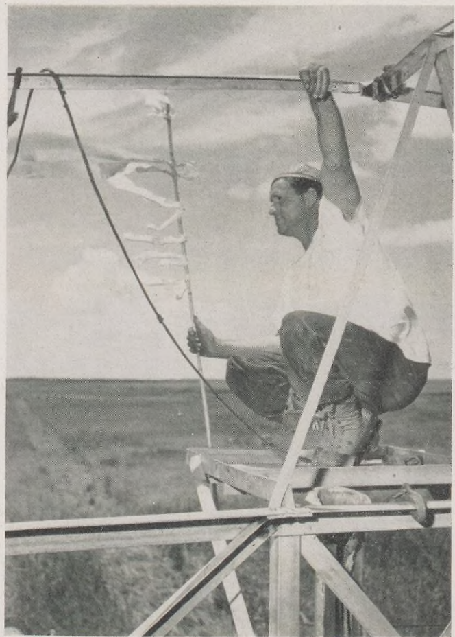
Traveling by helicopter and marsh buggy, surveyors are important members of exploration parties. Much of the marshland is unmapped and usual landmarks such as trees and shrubbery do not exist. Colored flags are set up (left) as targets for transit men who take readings on them to locate shot points. These are indicated by small, flagged stakes (being held by hand at right) to guide the members of the seismic party.
