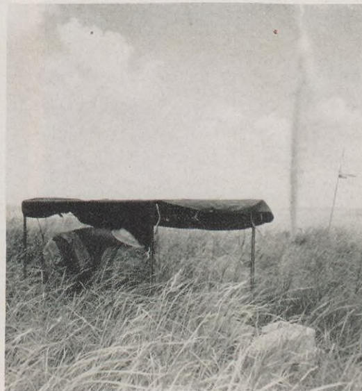
Sometimes the "shooter" (left) who sets off the charge, travels in a small wooden boat which is towed over the watery land behind the marsh buggy. He keeps in touch with other crew members by telephone. Ducking under his temporary shelter (center) the shooter fires the charge and mud and water fly up from the shot hole. After the shot, the operator checks a seismograph record (right) before moving to a new location.
