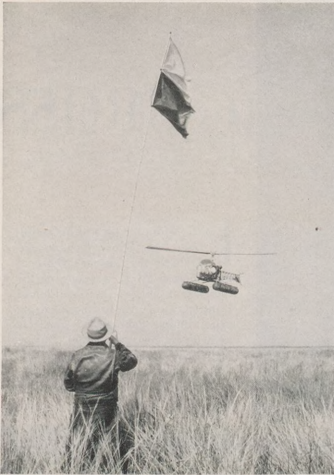
Traveling by helicopter and marsh buggy, surveyors are important members of exploration parties. Much of the marshland is unmapped and usual landmarks such as trees and shrubbery do not exist. Colored flags are set up (left) as targets for transit men who take readings on them to locate shot points. These are indicated by small, flagged stakes (being held by hand at right) to guide the members of the seismic party.
