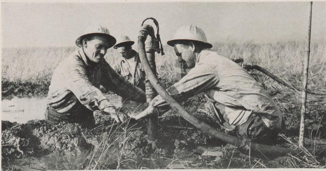
Up to their waists in muck, crew members complete the shot hole in the wet, boggy earth of the Louisiana marshland. The explosion to be detonated here will send out elastic waves which will be recorded by seismometers, giving clues to the structure of formations under the earth.
