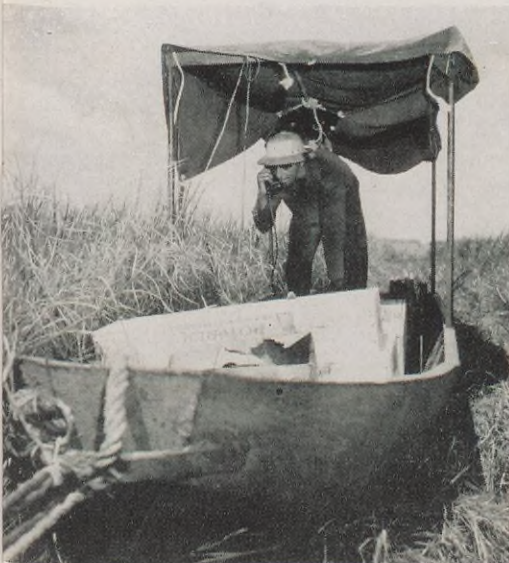
Sometimes the "shooter" (left) who sets off the charge, travels in a small wooden boat which is towed over the watery land behind the marsh buggy. He keeps in touch with other crew members by telephone. Ducking under his temporary shelter (center) the shooter fires the charge and mud and water fly up from the shot hole. After the shot, the operator checks a seismograph record (right) before moving to a new location.
