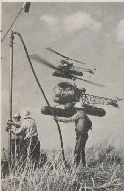
Pipe is assembled and forced into the earth by this shot hole drilling crew (left). Water is circulated through the hose to make drilling easier.
