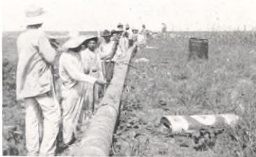
Applying Texaco felt covering
