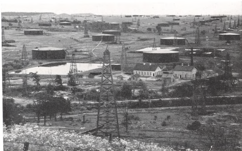
The Texas Company's Pump Station, Kiefer, Okla.
