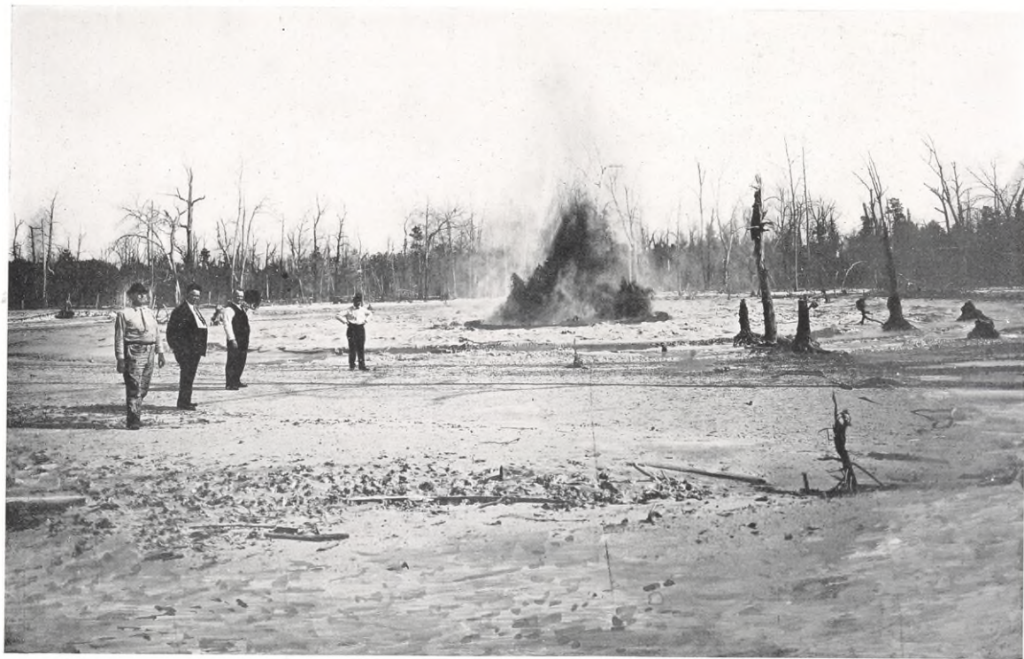
Dawes Trustee Well, Caddo Field—known as the "Wild Well," or the "Crater," showing the well spouting mud and water, and the crater formed around the well
