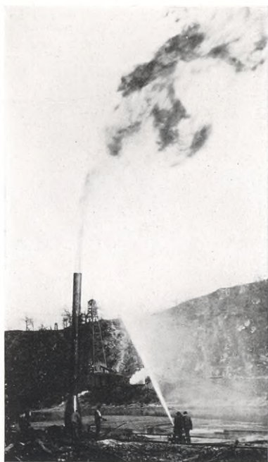
Hood placed on a burning gas well
