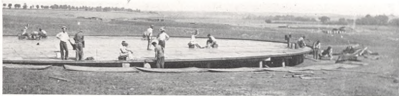
Laying bottom of a steel tank
