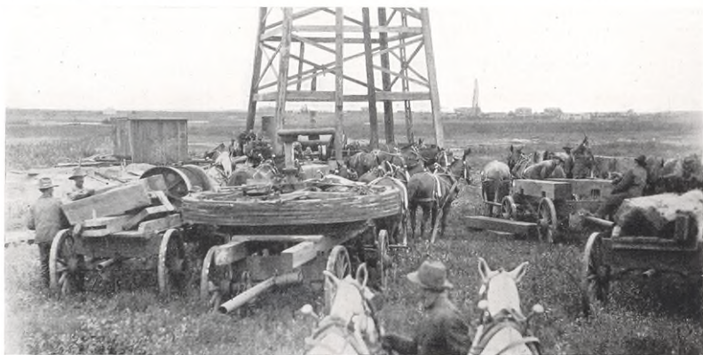
Standard rig parts being moved in to change rotary derrick to standard rig and derrick
