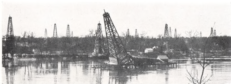
High water in Cimarron River—Cushing Field
