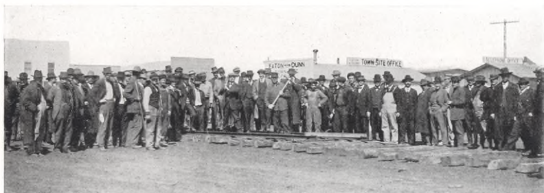
Driving the first spike at depot site, Oilton, March 23, 1915
