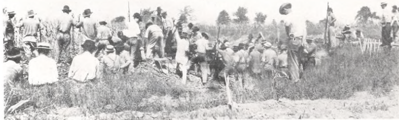
Crossing a gully—8" trunk line—loop south of Concord
