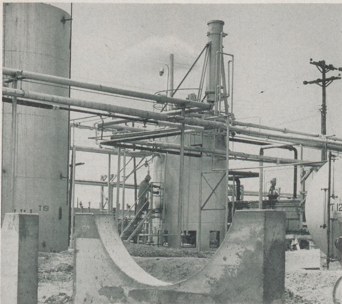
Part of an expansion program at the Denver Plant to meet the growing demand for Shell Chemical's three insecticides, the concrete saddles in foreground are ready for the installation of four 8,000-gallon storage tanks. Aldrin is made in the vertical reactor in the center background.
